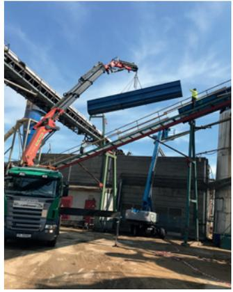
Photo: The new feedstock conveyor was produced at Forestia this summer, being installed during summer maintenance.
